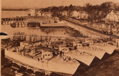
Each vessel in this quartet of PTs needs only one more torpedo tube. Then they will be ready to go over for the trial runs.
